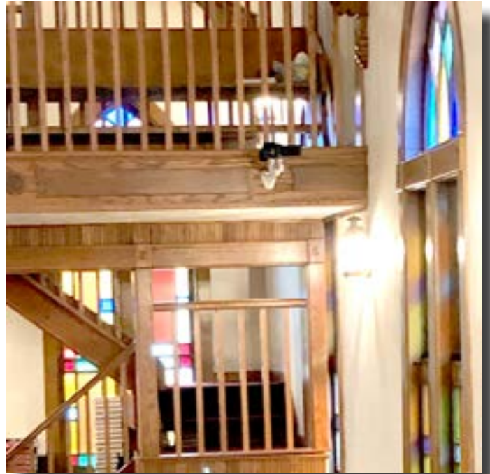
Video camera installed for live streaming church services
