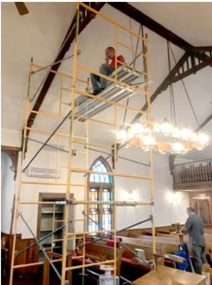
Technician from Buday Sound Advice installing audio equipment at CEC
